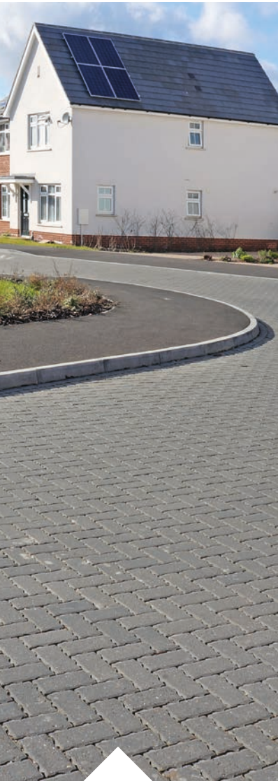
Concrete block permeable paving addresses both flooding and pollution by attenuating and cleaning water run-off at source. Peterborough City Council has trialled this approach at Fleetwood Crescent, a development for Cross Keys Homes. The drainage is designed to temporarily store rainwater run-off on site and remove pollutants before gradual discharge to a surface-water sewer that eventually outfalls into a nearby watercourse. House driveways and shared parking areas are also constructed in permeable paving, linked to the road construction with pipes below the footpath. Block paving supplied by Brett Landscaping.
